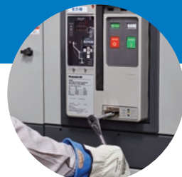
Levering Magnum DS breaker through the door
